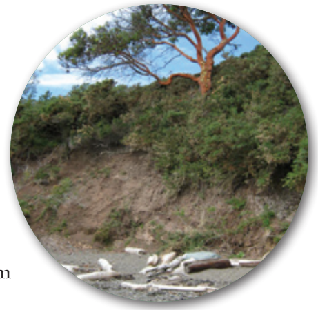
Above: Naturally eroding bluff
