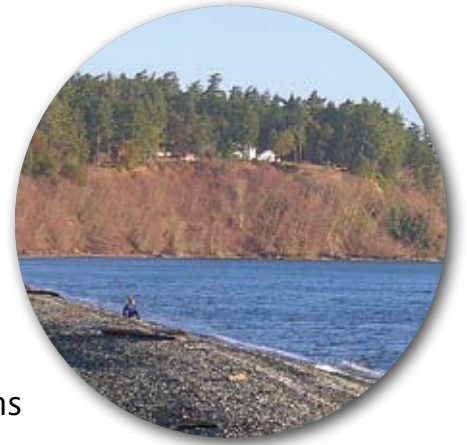
Above: Naturally eroding bluff
