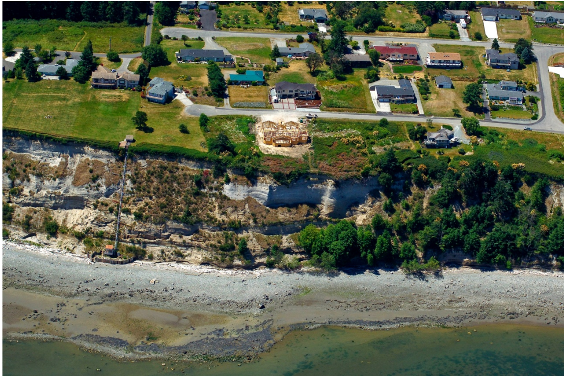
Figure 21. Air photo illustrating setbacks from the top of a bluff.
