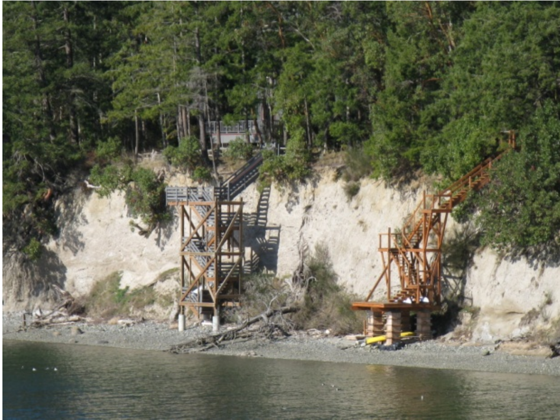
Figure 20. Stair towers on eroding bluff on Marrowstone Island.
