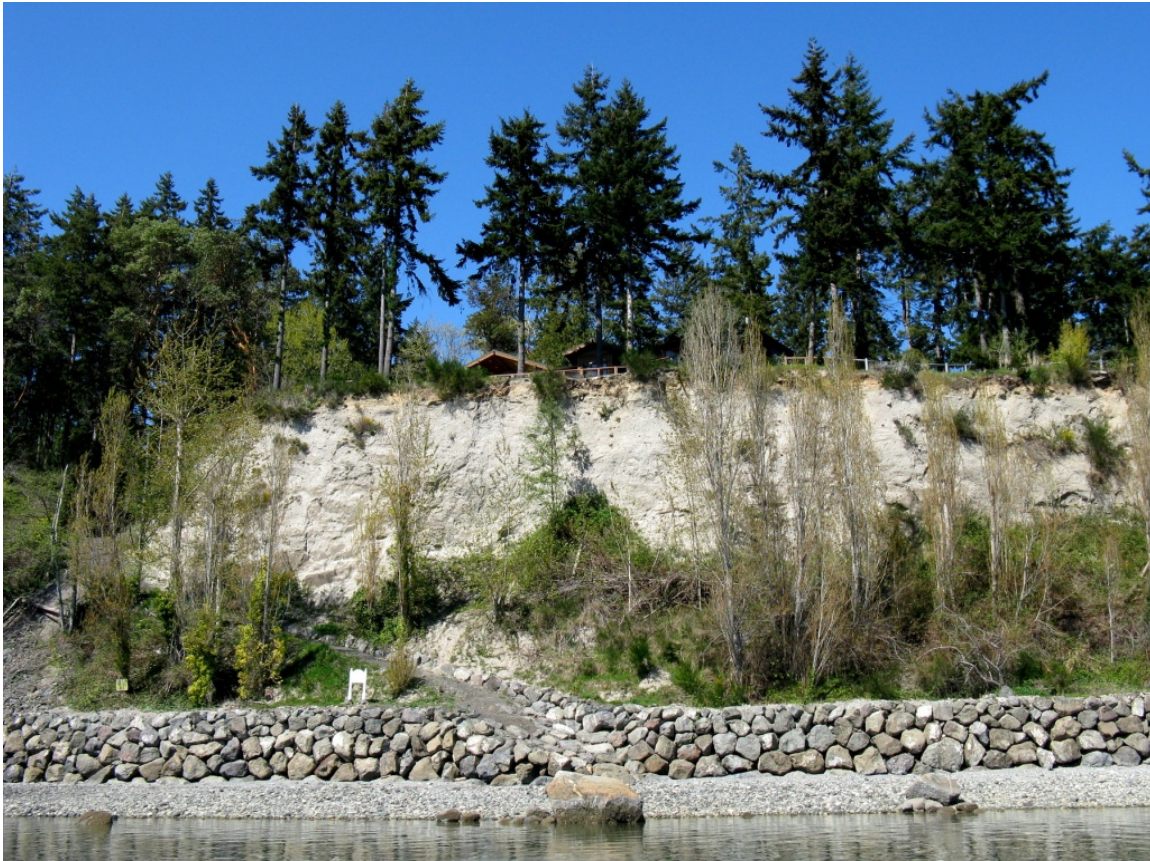
Figure 22. Rock bulkhead built to prevent erosion of bluff.
