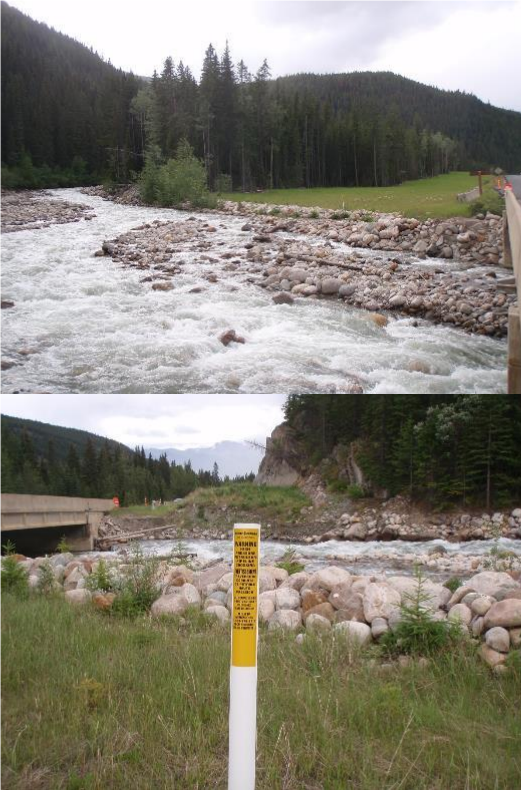
Figure 16 Extreme and unmitigated damage to the instream, bank and riparian areas for both stream-sides on Meadow Creek in Jasper National Park as a result of the TMP Anchor Loop project. Photo taken June 19, 2015.
