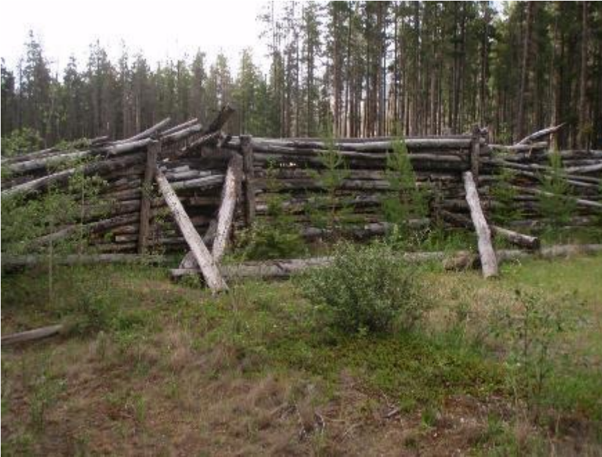
Figure 11 Large wooden structure located across the Anchor Loop corridor 2.6 km south of Snaring River. A number of these were constructed in the TMP ROW in Jasper National Park. Photo taken June 19, 2015.
