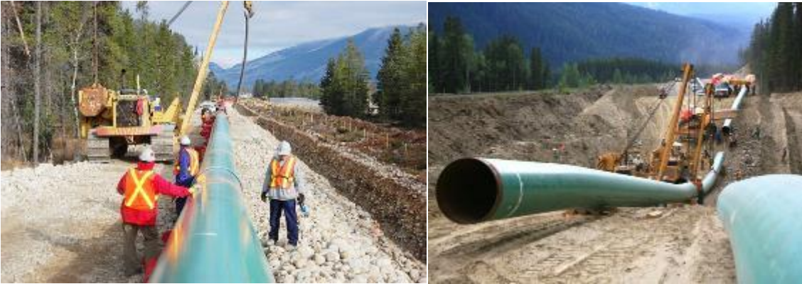
Figure 25 Large-scale ecological devastation of the landscape for both the existing ROW and construction zone when laying pipelines. When constructing petroleum pipelines, the vegetation is typically stripped in both the ROW and the construction zone, the landscape is compacted by machinery and all natural ecological function is destroyed. Left photo: http://www.vancouversun.com/business/things+know+about+Kinder+Morgan+pipeline+protest+Burnaby/10400385/story.html Right photo: https://financialpostcom.files.wordpress.com/2013/12/transmountain.jpg?w=620
