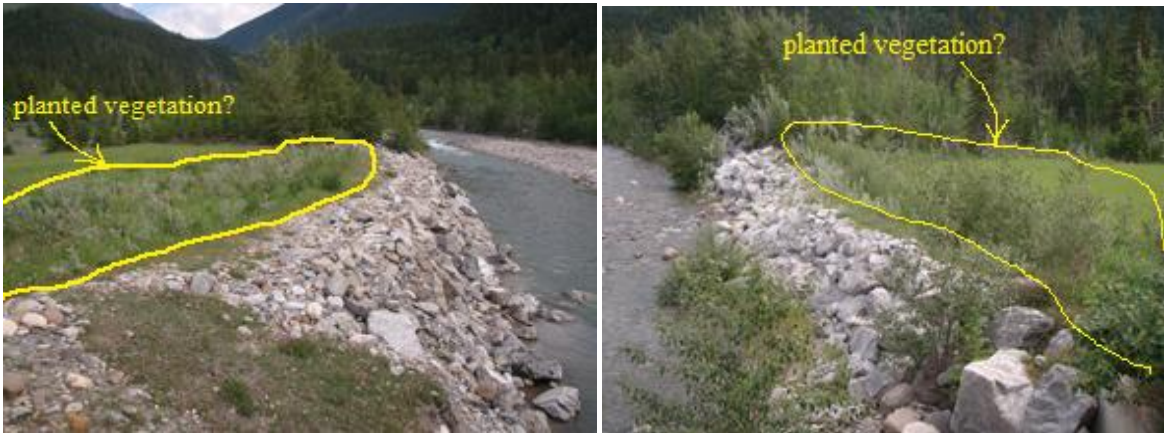
Figure 17 Right- (left photo) and left-bank (right photo) Fiddle River TMP crossing in the Jasper National Park section of the Anchor Loop project. Large-scale destruction of the shoreline integrity (riprapping) occurred here without any attempt at creating any instream or bank physical diversity. Unlike Meadow Creek, however, it appears that ~10 m of vegetation was planted along the riparian areas of this stream on both banks; nevertheless, it is clear that some of these shrubs/trees failed to properly survive and since 2008 most are only about knee-to-waist height (Figure 18).
