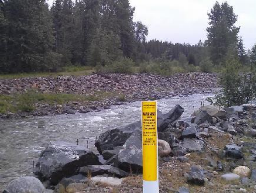
Figure 40 Extensive and extreme damage to the shoreline habitat of Juliet Creek on the Coldwater River drainage due to rip rapping, channelization and vegetation removal at the TMP crossing. Top photo: on left bank, looking downstream; Bottom photo: on left bank looking cross stream. Photos taken May 2015.
